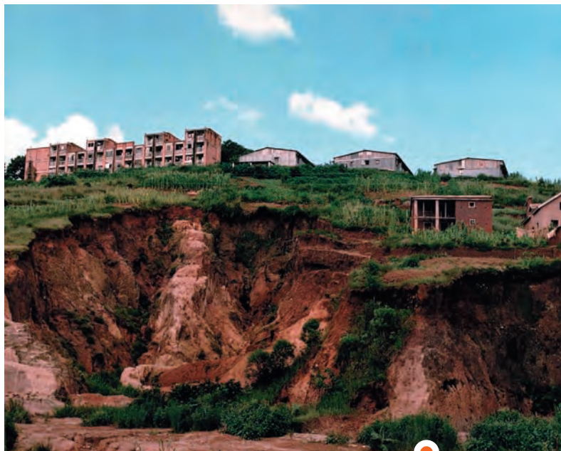
A scene from the "great red island" of Madagascar. On that island, the effects of deforestation, water runoff, and soil erosion are visible to the naked eye.
