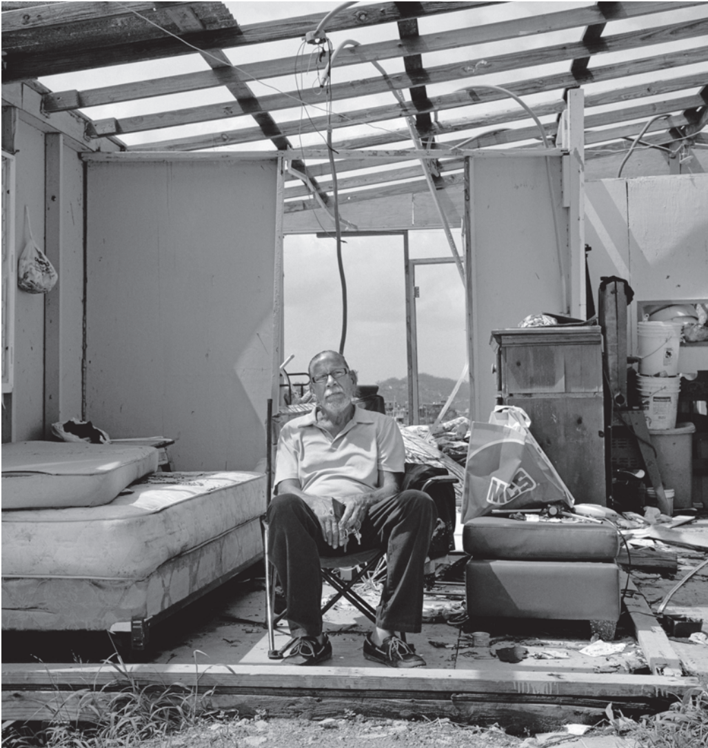
The gathering storm: at a house damaged by Hurricane Maria in Puerto Rico, October 2017
