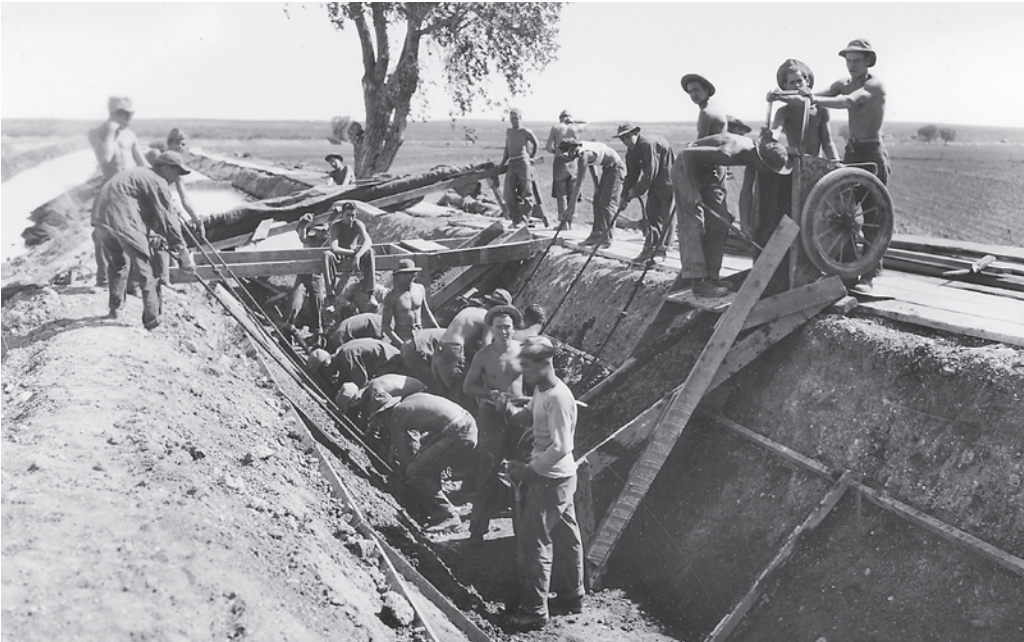
Fixing a hole: Civilian Conservation Corps workers lining a canal in New Mexico, 1940
