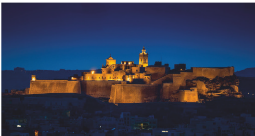
Gozo's historic Cittadella has been recently restored
