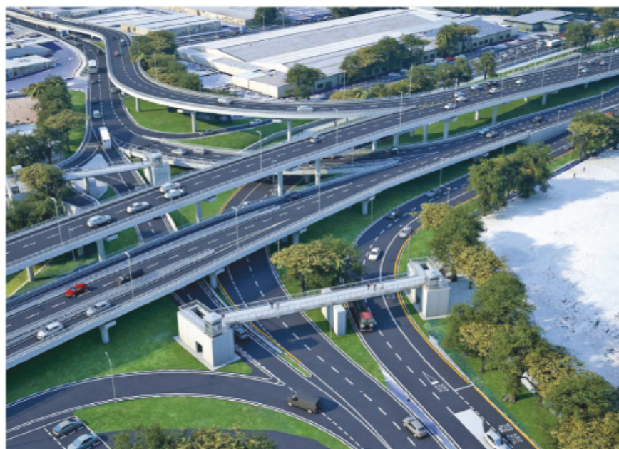
The government has committed itself to major road infrastructure projects
