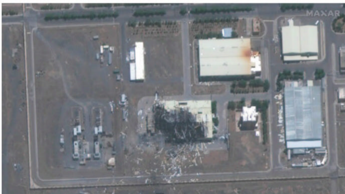
A shed-load of damage
