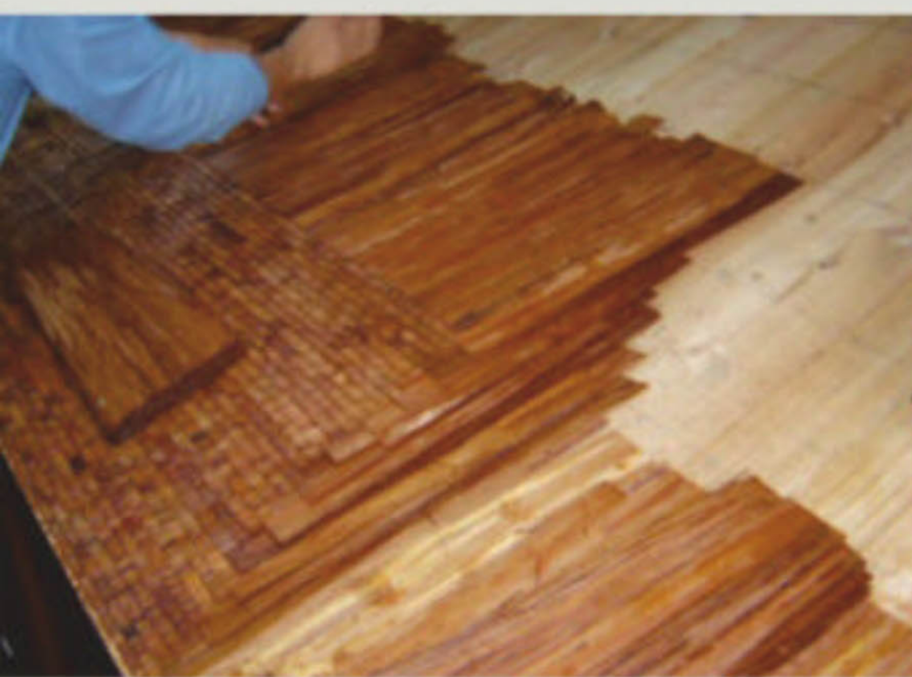
Hiwadabuki roof repair (cypress bark roofing).
