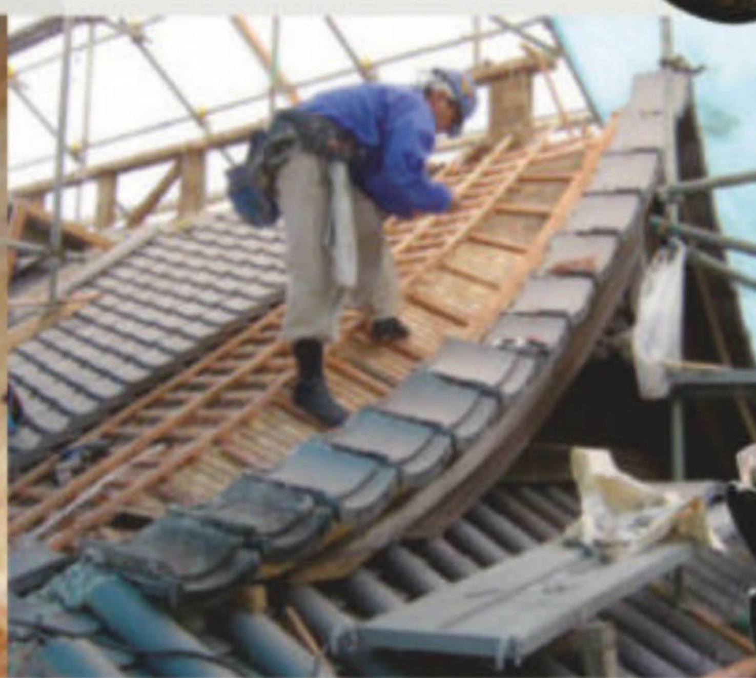
Hongawarabuki roof repair (formal tile roofing).
