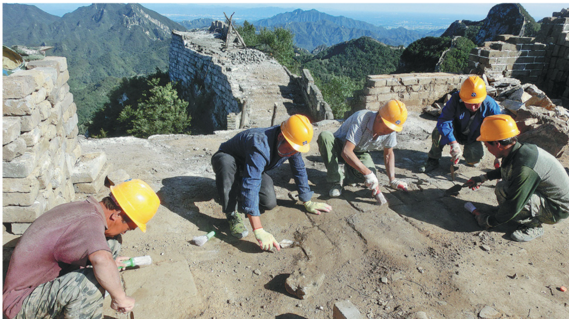
Workers clear the surface of the Jiankou section of the Great Wall to prepare for archaeological studies. PROVIDED TO CHINA DAILY
