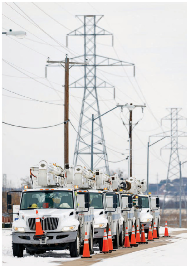
Electric service trucks line up in Fort Worth after a snowstorm leaves millions of Texans without power
