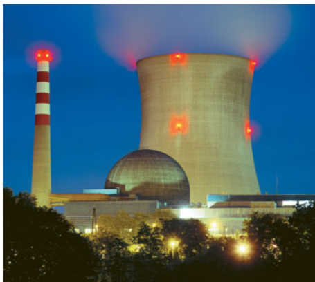
FIGURE 17.5 Comparison of (a) a fossil-fuel power plant and (b) a nuclear power plant with a boiling-water reactor. Notice that the nuclear reactor has exactly the same function as the boiler in the fossil-fuel power plant. The coal-burning plant (a) is Ratcliffe-on-Saw, in Nottinghamshire, England, and the nuclear power station (b) is in Leibstadt, Switzerland. (Source: American Nuclear Society, Nuclear Power and the Environment , 1973.)
