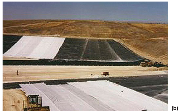
FIGURE 23.14 (a) Idealized diagram of a solid-waste facility (sanitary landfill) illustrating multiple-barrier design, monitoring system, and leachate collection system. (b) Rock Creek landfill under construction in Calaveras County, California. This municipal solid-waste landfill is underlain by a compacted clay liner, exposed in the center left portion of the photograph. The darker slopes, covered with gravel piles, overlie the compacted clay layer. These form a vapor barrier designed to keep moisture in the clay so it won't crack. Trenches at the bottom of the landfill are lined with plastic and are part of the leachate collection system for the landfill. The landfill is also equipped with a system to monitor the water below the leachate collection system.
