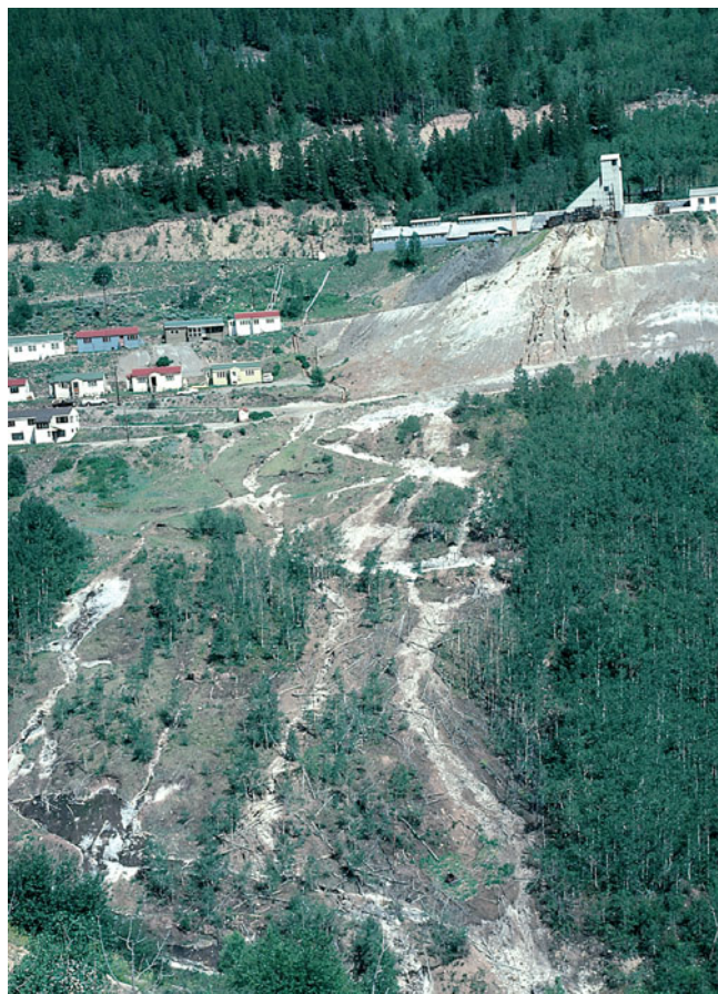
FIGURE 23.6 Tailings from a lead, zinc, and silver mine in Colorado. White streaks on the slope are mineral deposits apparently leached from the tailings.
