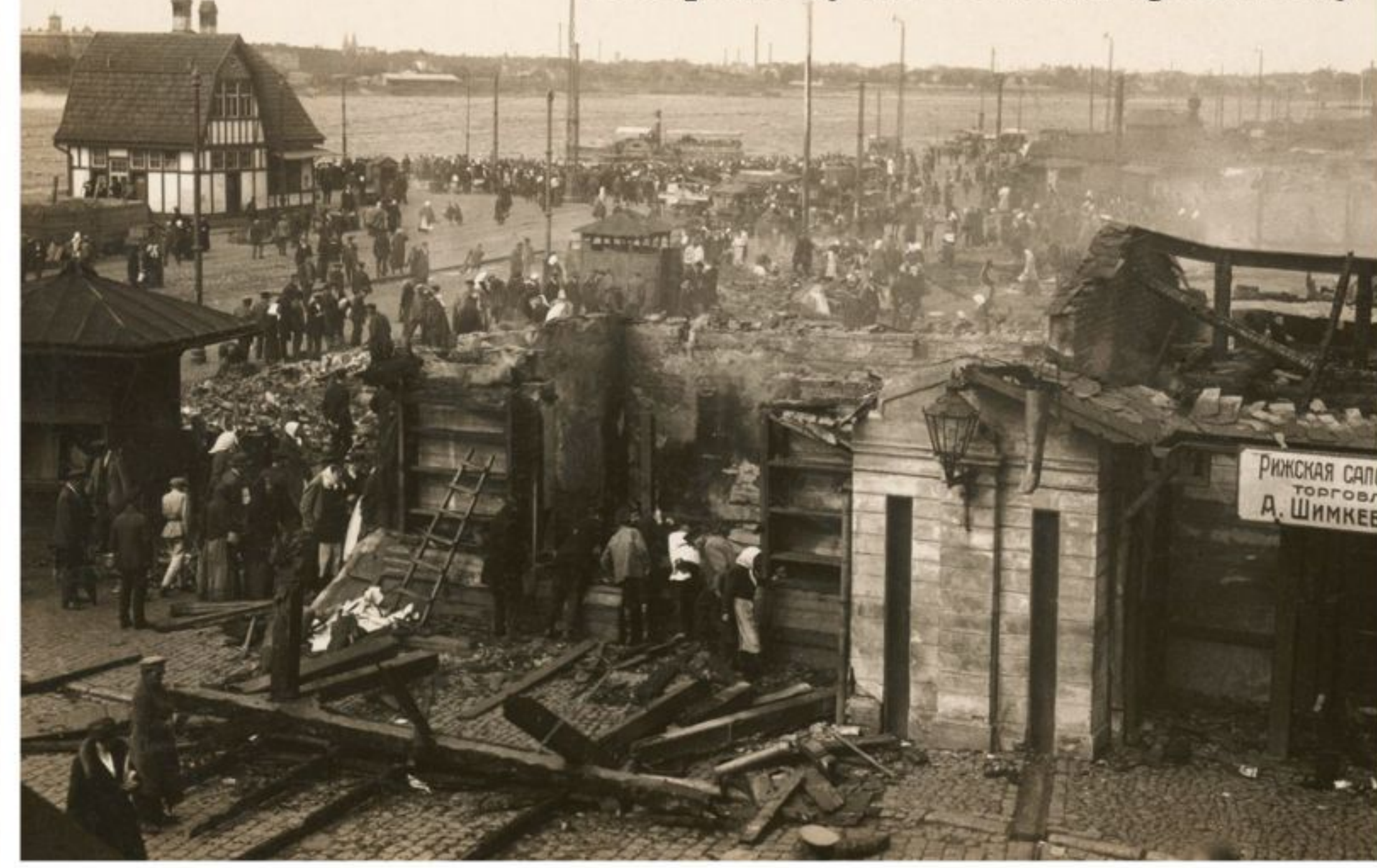
Damaged buildings in Riga, the capital city of Latvia, following its capture by the German Eighth Army
