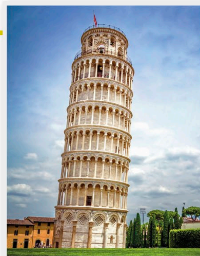
④ This Italian bell tower started to lean to one side in the soft ground during its construction, but has miraculously survived for more than 600 years!
