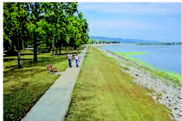
Figure 16.34 An example of engineered levees. This artificial levee along the Mississippi River in Guttenberg, Iowa, kept the Mississippi River from flooding the town during a minor flood in 2001. The U.S. Army Corps of Engineers built and maintains this structure, as well as many others like it, along the Mississippi.
