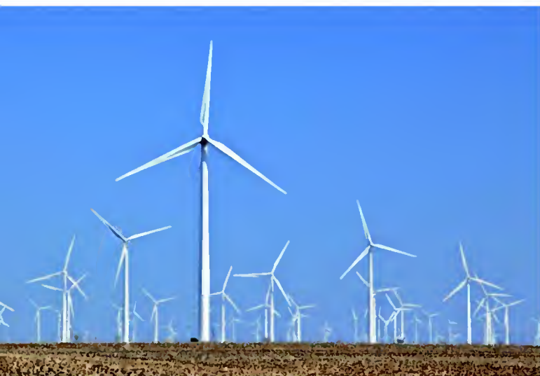
Figure 6.27 The Horse Hollow Wind Energy Center in Texas. This facility has over 400 turbines, which collectively produce enough energy for 220,000 homes per year.
