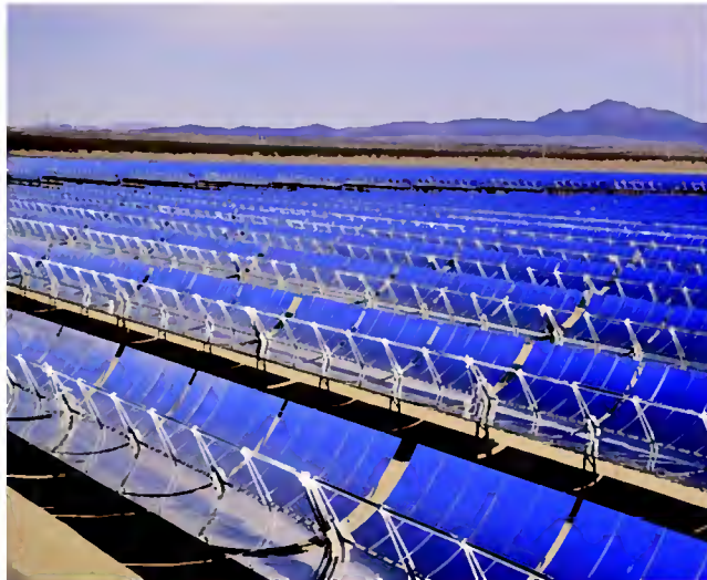
Figure 4.30 The Solar Energy Generating System in California's Mojave Desert. This photograph shows a portion of the complex. Over 936,000 trough energy collectors are contained within the entire system, producing enough electricity for 500,000 people per year.
