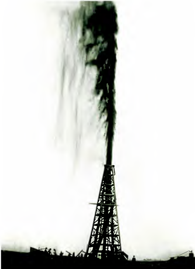
Figure 12.26 The Lucas gusher. In 1901 the Corsican oil field in southeastern Texas was tapped by Patillo Higgins, a self-taught geologist. The pressure in the well was so great that the oil (or “black gold”) erupted to a height of about 50 m (150 ft) for 9 days after the initial strike. Approximately 1,000,000 barrels of oil were lost, which would be worth about $17,000,000 today.
