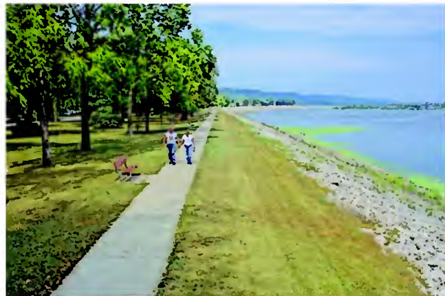
Figure 16.34 An example of engineered levees. This artificial levee along the Mississippi River in Guttenberg, Iowa, kept the Mississippi River from flooding the town during a minor flood in 2001. The U.S. Army Corps of Engineers built and maintains this structure, as well as many others like it, along the Mississippi.
