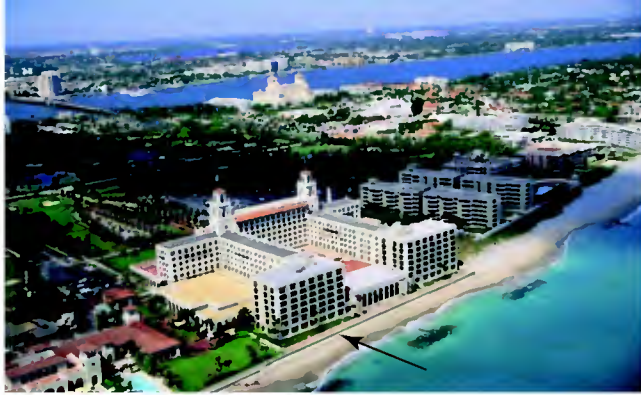
Figure 19.37 Sea walls. This sea wall (arrow) at Palm Beach, Florida, protects a hotel complex from coastal erosion. Structures like this armor much of the shore in southeastern Florida.
