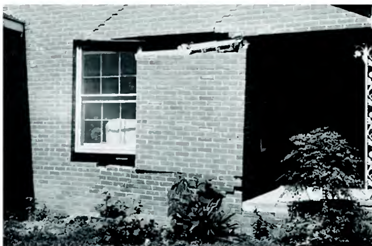
Figure 11.37 Cracked outside wall in a home built on clay-rich soils. This house was severely damaged because the surrounding soil contains expandable clays, which can either expand like a sponge when wet or lose cohesion and collapse when they dry.
