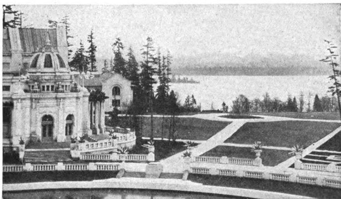
FIG. 184.—End of Manufacturers' Building, with Cascade Mountains in distance, Seattle.
