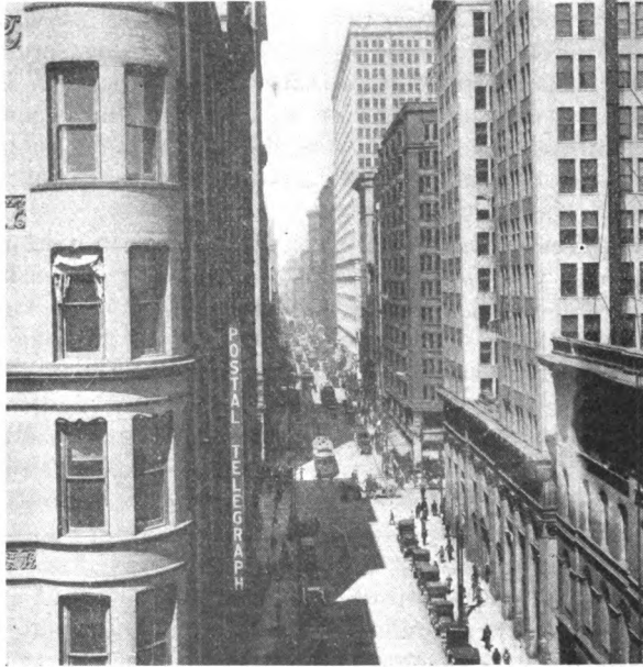
FIG. 170.—The Olive street canyon, St. Louis.
