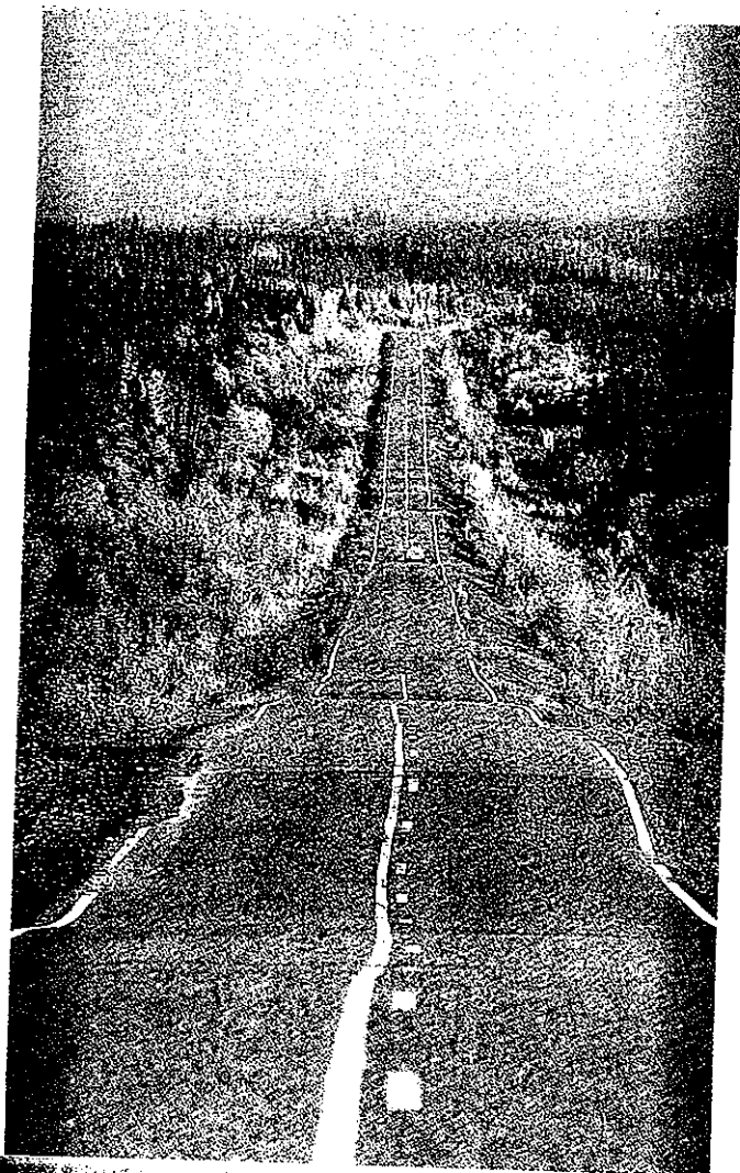
FIGURE 18-3 A once-smooth road after several annual cycles of freezing and thawing in the underlying surface layer of soil. This valley is located near Mt. Drum in south-central Alaska.
