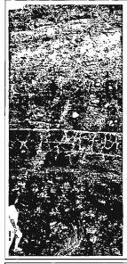
This road cutting in Hawaii shows an almost complete weathering sequence in basalt lavas.
