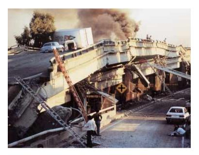
**Figure 10–9** Surface waves cause a large proportion of earthquake damage. Collapse of Interstate Highway 880 during the 1989 Loma Prieta, California, earthquake. (Paul Scott/Sygma)
