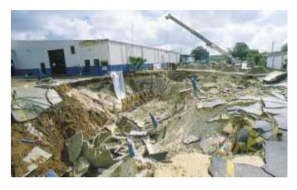
**Figure 15–11** A dropping water table caused subsidence and structural damage in Jacksonville, Florida. (Wendell Metzen/Bruce Coleman, Inc.)
