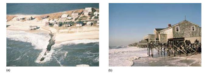
**Figure 18–22** (a) This aerial photograph of a Long Island beach shows sand accumulating on the upstream side of a groin, and erosion on the downstream side. (b) A closeup of the house in (a) shows waves lapping against the foundation.
