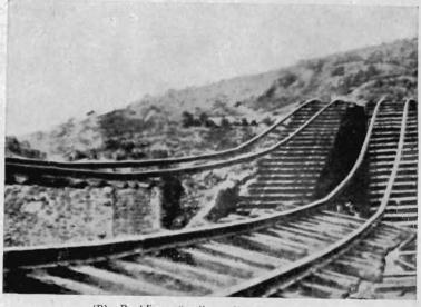
(B) Buckling of railway lines near Tokyo
