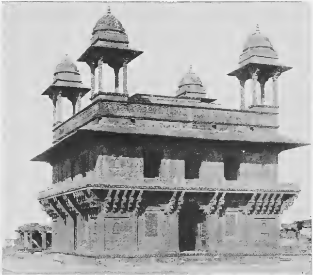
THE DIWAN-I-KHAS, FATHPUR-SIKRI.
