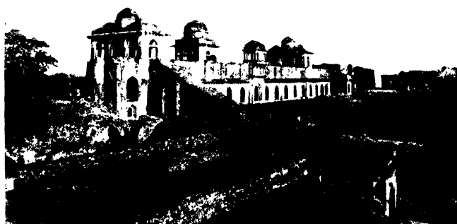
The Jahāz Mahall at Māndū
