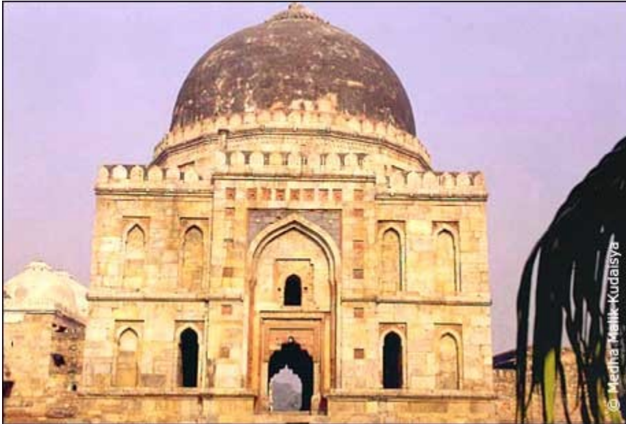
Bara Gumbad, constructed during the period of Lodhi Dynasty
