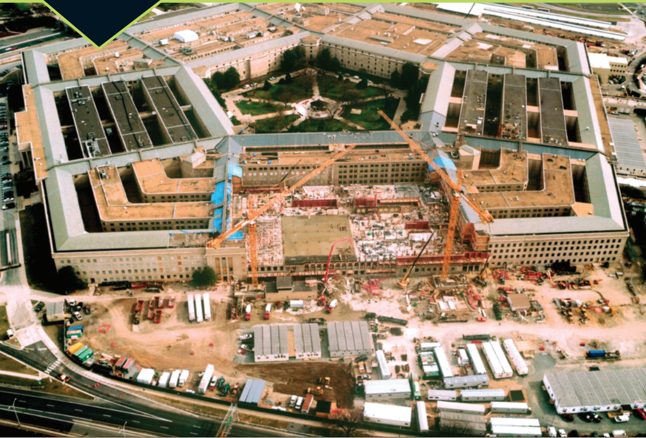
The Pentagon Rebuilds after the 9/11 Attack
