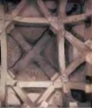
Left to right: Gothic type rib vaulting at Bab Mardum Mosque, built at the end of the 10 th century in Toledo, Spain; two examples of Gothic rib vaulting.
