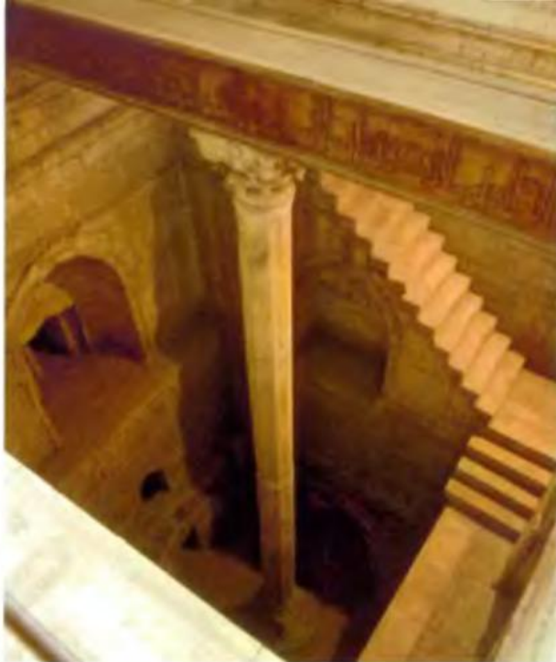
The nilometer in Rawada Island at Fustat, near Cairo, completed in 861-862 CE. The octagonal column in the centre is used to measure the height of the water in the Nile in cubits.
