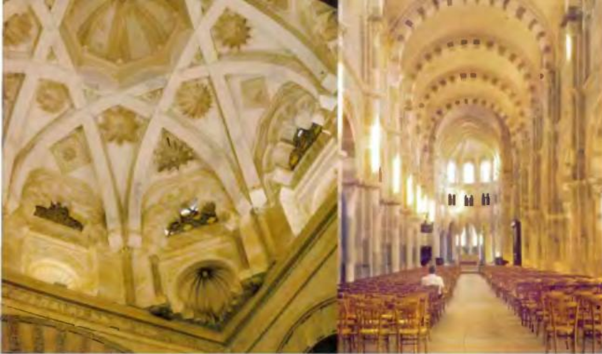
Left to right: Rib vaulting in the maqsura dome of the Great Mosque of Cordoba, added in the 10 th century; ribbed, tunnel vaults at 12 th -century Sainte-Madeleine in Vezelay, France, resembling those of Susa, built in 821–822.
