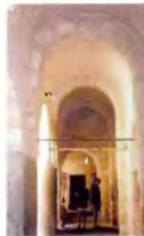
Ribs of the tunnel vaults of the Ribat of Susa, built in 821–822 CE.
