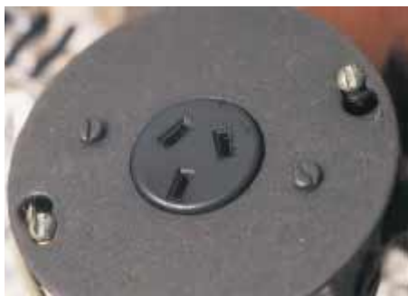
Figure 28.29 A power connection for a 240-V appliance.
