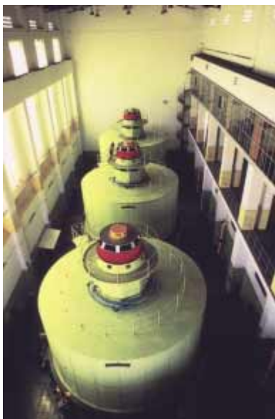
Turbines turn generators at a hydroelectric power plant. (Luis Casaneda/The Image Bank)
