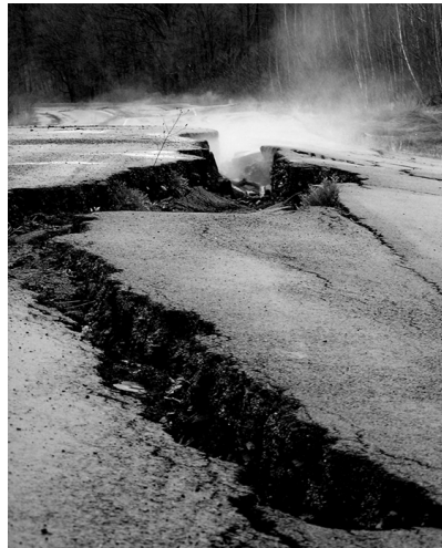
Figure 4.1: This underground mine fire in Centralia, Pennsylvania, could burn for over a century. (Photo courtesy of jesiehart/flickr)
