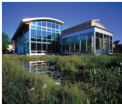
FIGURE 20.11 The Adam Joseph Lewis Center for Environmental Studies at Oberlin College is designed to be self-sustaining even in northern Ohio's cool, cloudy climate. Large, south-facing windows let in sunlight, while 370 m 2 of solar panels on the roof generate electricity. A constructed wetland outside and a living machine inside (see fig. 18.27) purify wastewater.
