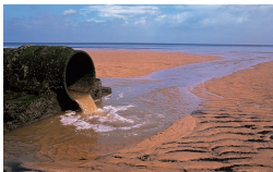
FIGURE 18.2 Sewer outfalls, industrial effluent pipes, acid draining out of abandoned mines, and other point sources of pollution are generally easy to recognize.
