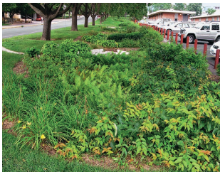
FIGURE 18.28 A rain garden is a shallow depression situated to collect runoff from streets or parking lots. It's planted with species that can survive in saturated soils. This vegetation helps evaporate and cleanse runoff, while temporary storage in the basin allows groundwater recharge. You might build a rain garden in your yard, or on your campus, or elsewhere in your city.
