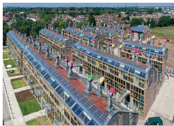
South-facing windows heat homes, and colorful, rotating "wind cowls" ventilate rooms at BedZED , an ecological housing complex in South London, U.K.
