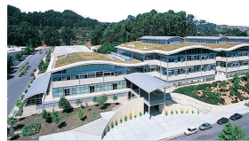
FIGURE 23.26 The award-winning Gap, Inc. corporate offices in San Bruno, California, demonstrate some of the best features of environmental design. A roof covered with native grasses provides insulation and reduces runoff. Natural lighting, an open design, and careful relation to its surroundings all make this a pleasant place to work.
