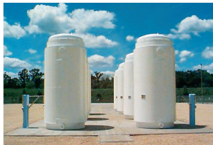
FIGURE 19.26 Spent fuel is being stored temporarily in large, aboveground "dry casks" at many nuclear power plants.
