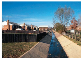
FIGURE 13.29 Many former streams have been turned into concrete-lined ditches to control erosion and speed runoff. The result is an artificial system with little resemblance to the living biological community that once made up the stream.
