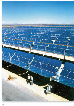
FIGURE 20.13 Concentrating solar power (CSP) uses either mirrored troughs (a) or movable mirrors focused on a central tower (c) to generate steam that turns a turbine to generate electricity. Often these facilities are sited in deserts where sunshine is intense and land is unoccupied. Large industrial facilities can intrude, however, on desert wildlife, solitude, and beauty (b).
