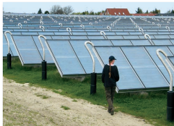
FIGURE 20.12 Solar water heaters can be scaled up to provide hot water and space heating for whole cities.
