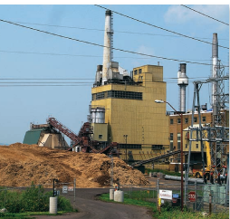
FIGURE 20.18 This Michigan power plant uses wood chips to fuel its boilers. Where wood supplies are nearby, this is a good choice both economically and environmentally.
