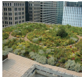
FIGURE 22.19 This award-winning green roof on the Chicago City Hall is functional as well as beautiful. It reduces rain runoff by about 50 percent, and keeps the surface as much as 30°F cooler than a conventional roof on hot summer days.
