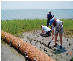
FIGURE 13.26 Volunteers plant dune grasses as part of Chesapeake Bay restoration. The large cylinder is a “bio log” made of biodegradable material that will help stabilize the shore.
