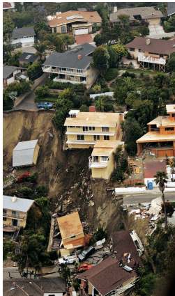
FIGURE 14.22 Damaged homes sit on a hillside after a landslide in Laguna Beach, Calif.
