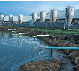
FIGURE 9.14 This state-of-the-art lagoon is built to store manure from a hog farm. Odors and overflow after storms are risks of open lagoons, but more thorough waste treatment is expensive.
