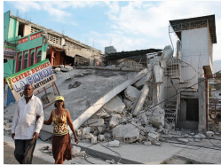
FIGURE 14.18 Earthquakes are most devastating where building methods can't withstand shaking. The 2010 earthquake in Haiti is thought to have killed 230,000 people. Collapsed buildings, food and water shortages, infectious diseases, and exposure to the elements all contributed to the death toll.
