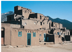
FIGURE 20.10 Taos Pueblo in northern New Mexico uses adobe construction to keep warm at night and cool during the day.
