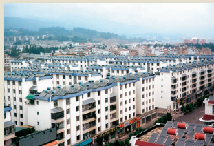
FIGURE 1.1 China already has more than 40 million rooftop solar collectors and has recently become the world's leader in renewable energy.
