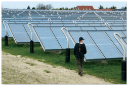
FIGURE 20.12 Solar water heaters can be scaled up to provide hot water and space heating for whole cities.
