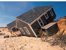
FIGURE 5.19 Winter storms have eroded the beach and undermined the foundations of homes on this barrier island. Breaching through protective dunes to build such houses damages sensitive plant communities and exposes the whole island to storms and erosion. Coastal zone management attempts to limit development on fragile sites.
