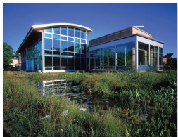
FIGURE 20.11 The Adam Joseph Lewis Center for Environmental Studies at Oberlin College is designed to be self-sustaining even in northern Ohio's cool, cloudy climate. Large, south-facing windows let in sunlight, while 370 m 2 of solar panels on the roof generate electricity. A constructed wetland outside and a living machine inside (see fig. 18.27) purify wastewater.
