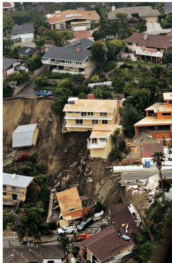
FIGURE 14.22 Damaged homes sit on a hillside after a landslide in Laguna Beach, Calif.
