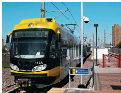
FIGURE 22.16 Many American cities are now rebuilding light rail systems that were abandoned in the 1950s when freeways were built. Light rail is energy-efficient and popular, but it can cost up to $100 million per mile ($60 million per kilometer).
