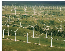
FIGURE 20.28 Wind is the fastest growing power source in the United States and represented more than 40 percent of new installed capacity in 2010.
