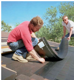
(a) Flexible, thin-film solar tiles
