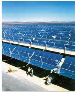
FIGURE 20.13 Concentrating solar power (CSP) uses either mirrored troughs (a) or movable mirrors focused on a central tower (c) to generate steam that turns a turbine to generate electricity. Often these facilities are sited in deserts where sunshine is intense and land is unoccupied. Large industrial facilities can intrude, however, on desert wildlife, solitude, and beauty (b).
