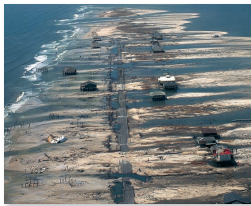
FIGURE 14.24 The aftermath of Hurricane Katrina on Dauphin Island, Alabama. Since 1970 this barrier island at the mouth of Mobile Bay has been overwashed at least five times. More than 20 million yd 3 (15 million m 3 ) of sand has been dredged or trucked in to restore the island. Some beach houses have been rebuilt, mostly at public expense, five times. Does it make sense to keep rebuilding in such an exposed place?
