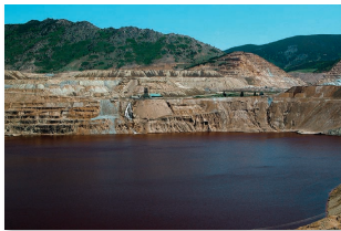
FIGURE 13.34 The Berkeley mine pit in Butte, Montana, may be the most toxic water body in the United States. Water entering the pit is now being treated and eventually there may be an effort to pump water out of the pit and decontaminate it, but the pit itself will probably never be filled in.
