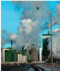
FIGURE 16.6 The most annoying pollutants from this paper mill are pungent organosulfur thiols and sulfides. Chlorine bleaching can also produce extremely dangerous organochlorines, such as dioxins.
