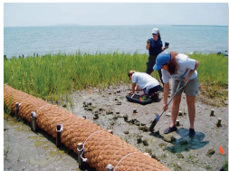
FIGURE 13.26 Volunteers plant dune grasses as part of Chesapeake Bay restoration. The large cylinder is a “bio log” made of biodegradable material that will help stabilize the shore.
