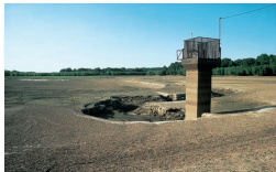
FIGURE 17.21 This dam is now useless because its reservoir has filled with silt and sediment.
