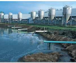
FIGURE 9.14 This state-of-the-art lagoon is built to store manure from a hog farm. Odors and overflow after storms are risks of open lagoons, but more thorough waste treatment is expensive.
