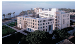
FIGURE 25.13 The University of California at Santa Barbara claims its new Bren School of Environmental Science and Management is the most environmentally friendly building of its kind in the United States.
