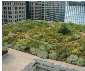
FIGURE 22.19 This award-winning green roof on the Chicago City Hall is functional as well as beautiful. It reduces rain runoff by about 50 percent, and keeps the surface as much as 30°F cooler than a conventional roof on hot summer days.
