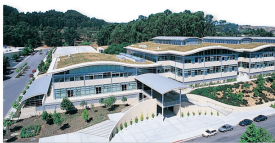
FIGURE 23.26 The award-winning Gap, Inc. corporate offices in San Bruno, California, demonstrate some of the best features of environmental design. A roof covered with native grasses provides insulation and reduces runoff. Natural lighting, an open design, and careful relation to its surroundings all make this a pleasant place to work.
