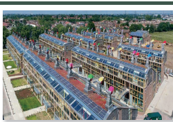
South-facing windows heat homes, and colorful, rotating "wind cows" ventilate rooms at BedZED, an ecological housing complex in South London, U.K.
