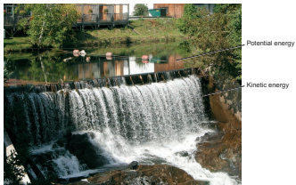
FIGURE 3.8 Water stored behind this dam represents potential energy. Water flowing over the dam has kinetic energy, some of which is converted to heat.
