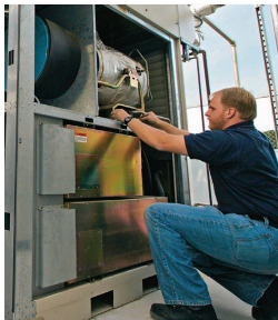
FIGURE 20.8 A technician adjusts a gas microturbine that produces on-site heat and electricity for businesses, industry, or multiple housing units.
