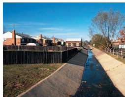
FIGURE 13.29 Many former streams have been turned into concrete-lined ditches to control erosion and speed runoff. The result is an artificial system with little resemblance to the living biological community that once made up the stream.
