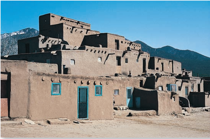
FIGURE 20.10 Taos Pueblo in northern New Mexico uses adobe construction to keep warm at night and cool during the day.
