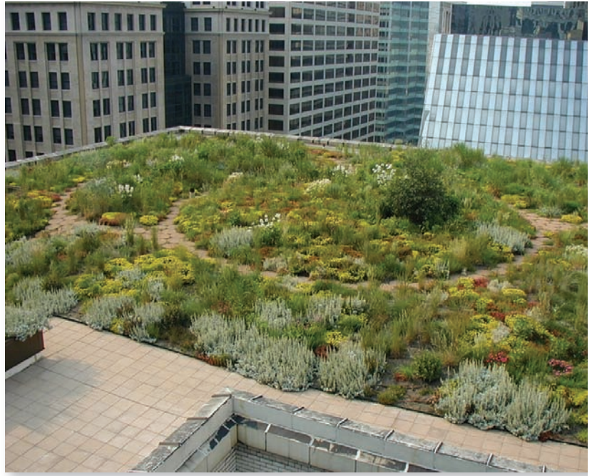
FIGURE 22.19 This award-winning green roof on the Chicago City Hall is functional as well as beautiful. It reduces rain runoff by about 50 percent, and keeps the surface as much as 30°F cooler than a conventional roof on hot summer days.
