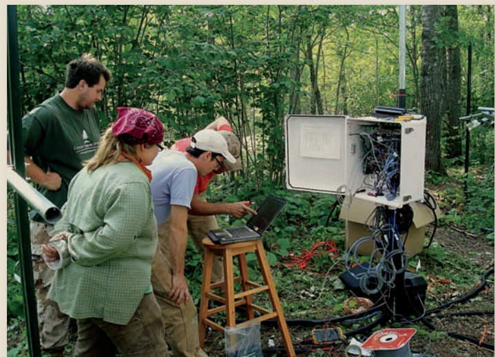
FIGURE 2.2 A student researcher adjusts the electrical panel that controls heat lamps and heating cables.
