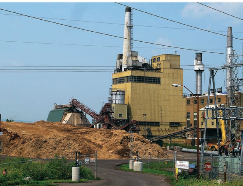
FIGURE 20.18 This Michigan power plant uses wood chips to fuel its boilers. Where wood supplies are nearby, this is a good choice both economically and environmentally.
