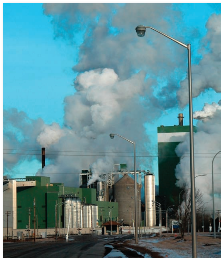
FIGURE 16.6 The most annoying pollutants from this paper mill are pungent organosulfur thiols and sulfides. Chlorine bleaching can also produce extremely dangerous organochlorines, such as dioxins.
