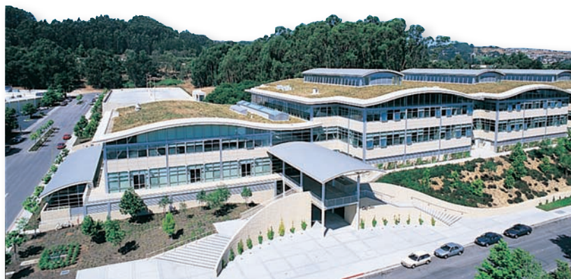
FIGURE 23.26 The award-winning Gap, Inc. corporate offices in San Bruno, California, demonstrate some of the best features of environmental design. A roof covered with native grasses provides insulation and reduces runoff. Natural lighting, an open design, and careful relation to its surroundings all make this a pleasant place to work.
