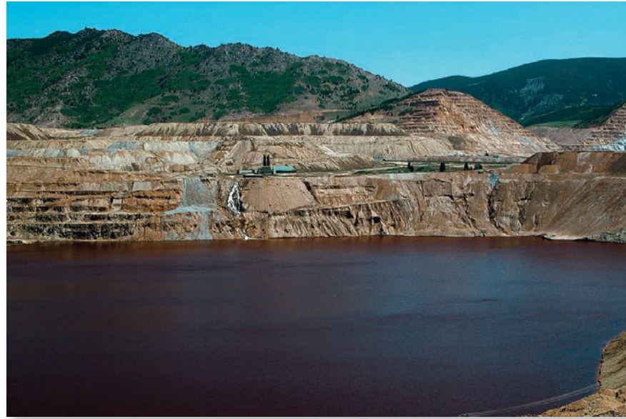
FIGURE 13.34 The Berkely mine pit in Butte, Montana, may be the most toxic water body in the United States. Water entering the pit is now being treated and eventually there may be an effort to pump water out of the pit and decontaminate it, but the pit itself will probably never be filled in.
