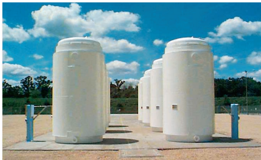
FIGURE 19.26 Spent fuel is being stored temporarily in large, aboveground “dry casks” at many nuclear power plants.
