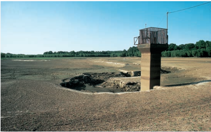
FIGURE 17.21 This dam is now useless because its reservoir has filled with silt and sediment.
