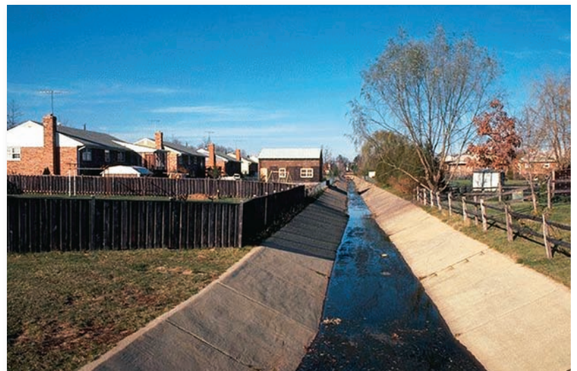
FIGURE 13.29 Many former streams have been turned into concrete-lined ditches to control erosion and speed runoff. The result is an artificial system with little resemblance to the living biological community that once made up the stream.
