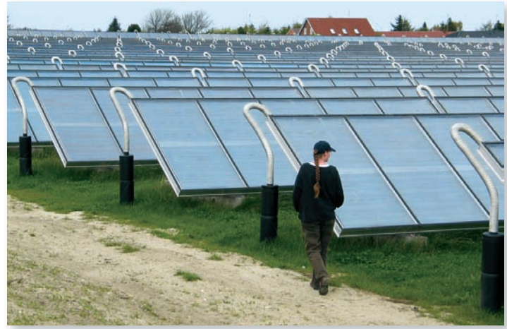
FIGURE 20.12 Solar water heaters can be scaled up to provide hot water and space heating for whole cities.
