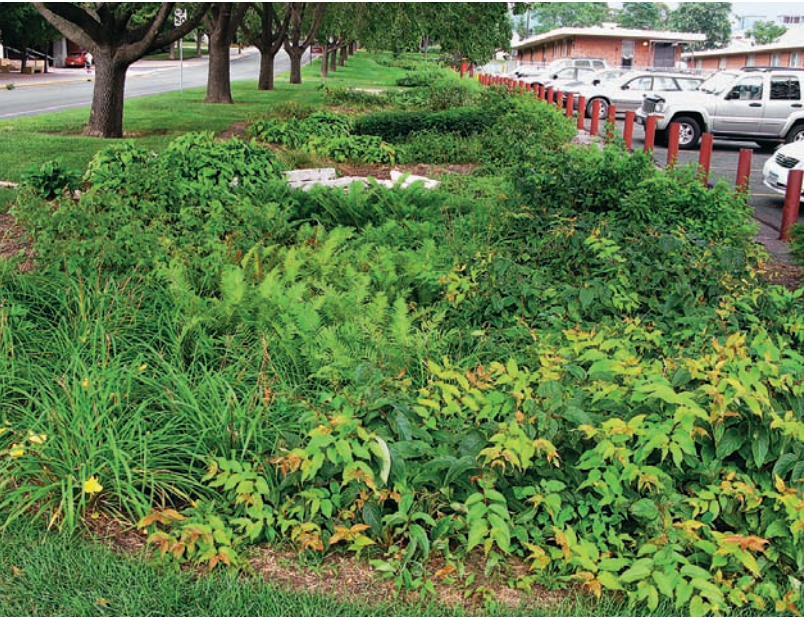
FIGURE 18.28 A rain garden is a shallow depression situated to collect runoff from streets or parking lots. It's planted with species that can survive in saturated soils. This vegetation helps evaporate and cleanse runoff, while temporary storage in the basin allows groundwater recharge. You might build a rain garden in your yard, or on your campus, or elsewhere in your city.
