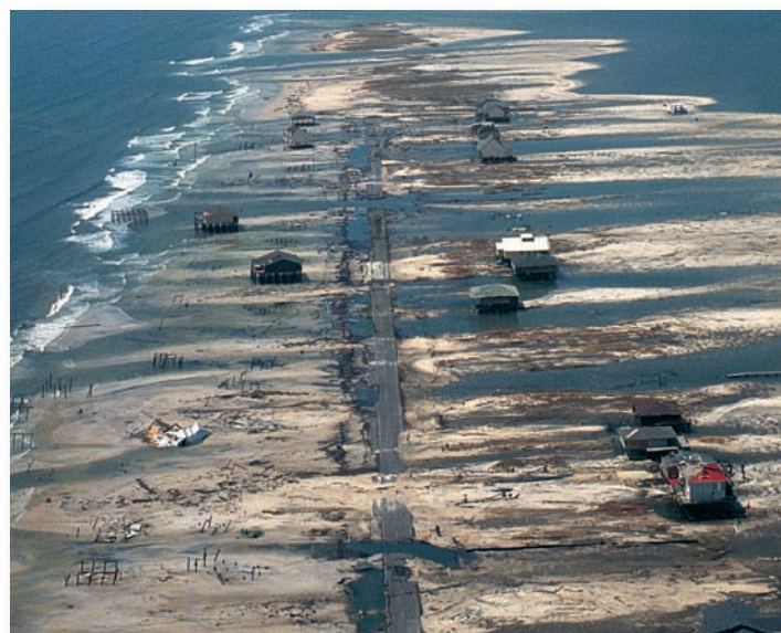
FIGURE 14.24 The aftermath of Hurricane Katrina on Dauphin Island, Alabama. Since 1970 this barrier island at the mouth of Mobile Bay has been overwashed at least five times. More than 20 million yd 3 (15 million m 3 ) of sand has been dredged or trucked in to restore the island. Some beach houses have been rebuilt, mostly at public expense, five times. Does it make sense to keep rebuilding in such an exposed place?
