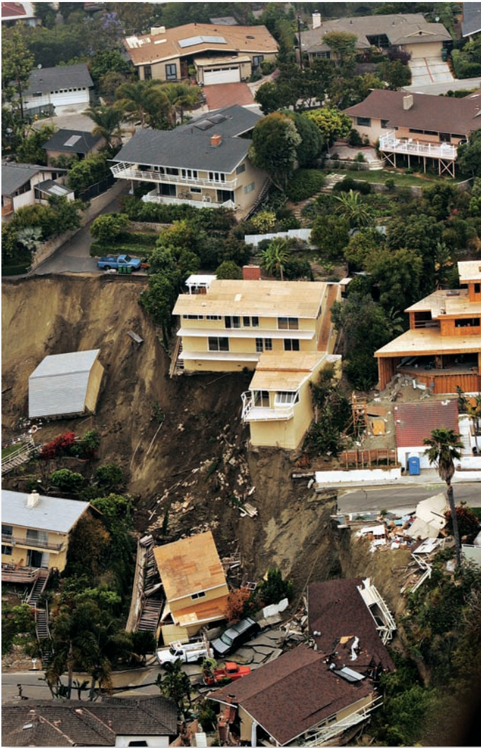
FIGURE 14.22 Damaged homes sit on a hillside after a landslide in Laguna Beach, Calif.
