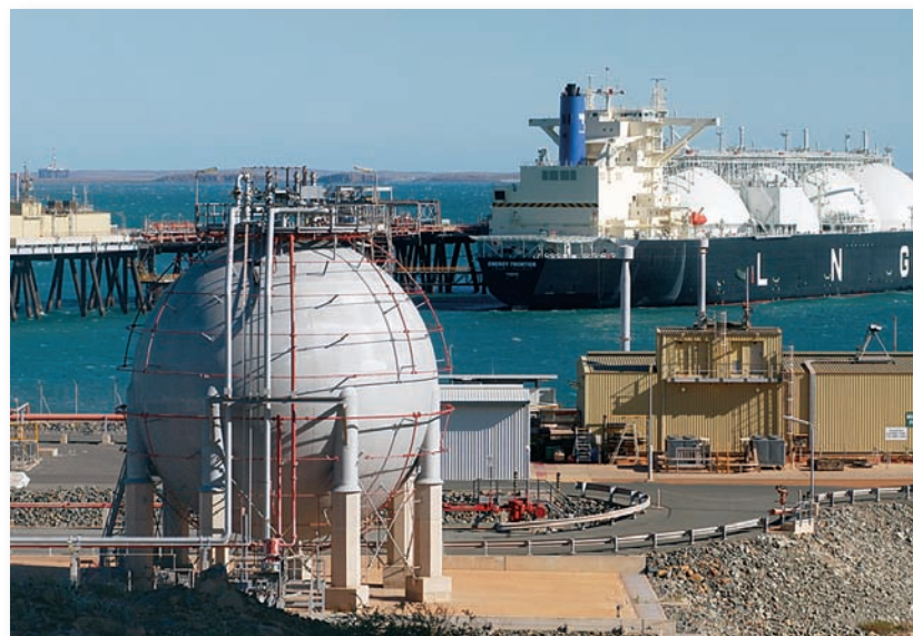
FIGURE 19.19 As domestic supplies of natural gas dwindle, the United States is turning increasingly to shipments of liquefied gas in specialized ships, such as this one at an Australian terminal. An explosion of one of these ships would release about as much energy as a medium-size atomic bomb.
