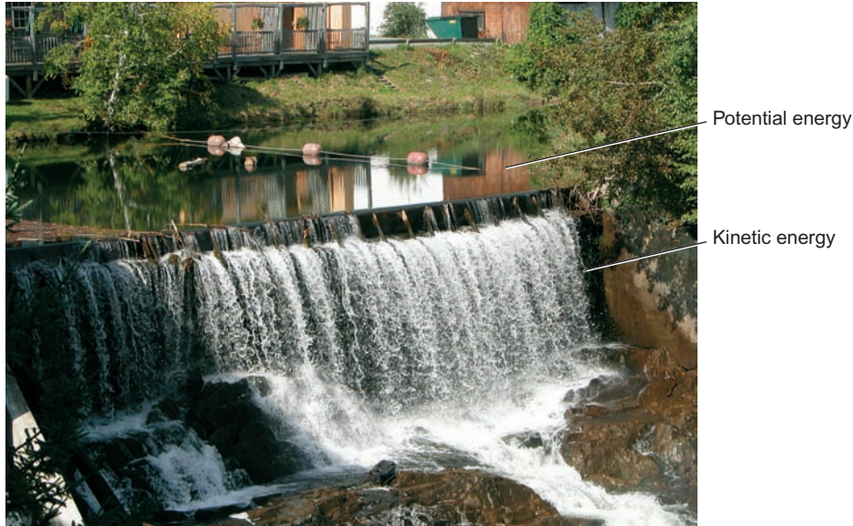
FIGURE 3.8 Water stored behind this dam represents potential energy. Water flowing over the dam has kinetic energy, some of which is converted to heat.
