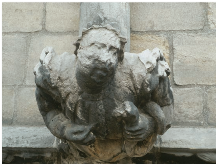
FIGURE 16.23 Atmospheric acids, especially sulfuric and nitric acids, have almost completely eaten away the face of this medieval statue. Each year the total loss from air pollution damage to buildings and materials amounts to billions of dollars.
