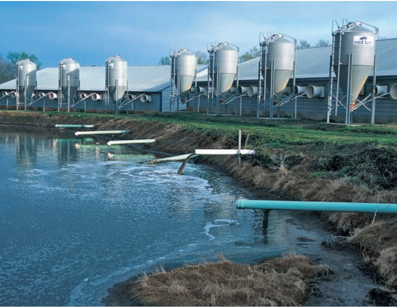
FIGURE 9.14 This state-of-the-art lagoon is built to store manure from a hog farm. Odors and overflow after storms are risks of open lagoons, but more thorough waste treatment is expensive.
