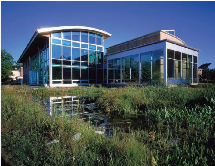
FIGURE 20.11 The Adam Joseph Lewis Center for Environmental Studies at Oberlin College is designed to be self-sustaining even in northern Ohio's cool, cloudy climate. Large, south-facing windows let in sunlight, while 370 \text{ m}^2 of solar panels on the roof generate electricity. A constructed wetland outside and a living machine inside (see fig. 18.27) purify wastewater.
